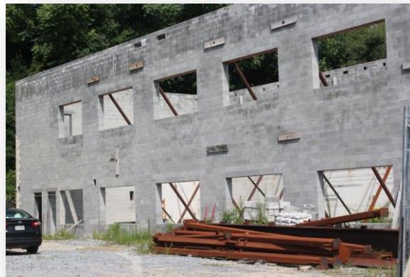
August 2016 photographs of LIUNA Local 657 training center in Washington, DC, left unfinished due to embezzlement of more than $1.7 million in union funds
